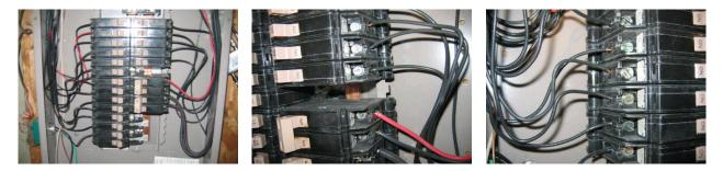
The system does not include arc-fault circuit interrupters, which effective January 1st, 2002, are mandated by the national electrical code to protect 15 and 20 amp branch circuits serving bedrooms in new construction. This is not a new home, so simply consider the benefit of installing them.
