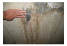
There are dry water marks around the sewer line. Located on the front wall.
