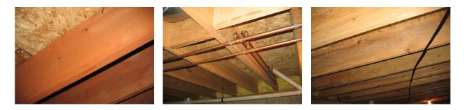
There have been structural repairs to floor under front entry door. Ask seller about prior repairs and possible water penetration problems.
