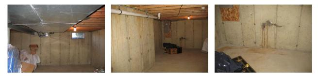
There is insulation at the band or rim joist areas, which is above the foundation wall, at the outer perimeter of the floor system. This insulation restricts the visual inspection of those areas considerably.
