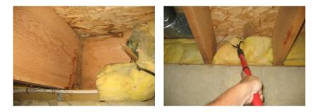
The floor joists are made of dimensional wood lumber - 2x10s.
