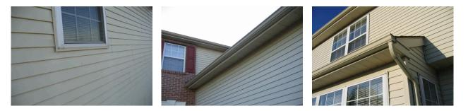
The vinyl siding appears functional. No major damage or deterioration was apparent. Recommend monitoring during a rain storm to see how the siding repels water. Be sure that the places where siding meets a different material is sealed or water-tight.
