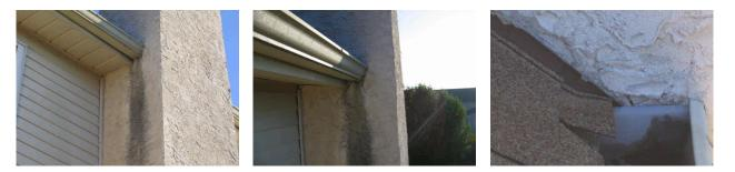
Major water damage visible from basement under the fireplace. Apparently caused by the missing flashing. Further evaluation of the structural integrity of the stack is recommended.
